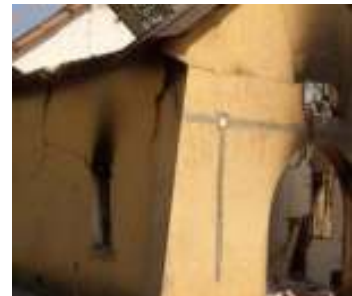
Radio house at Garamba NP HQ – before & after RRF support
